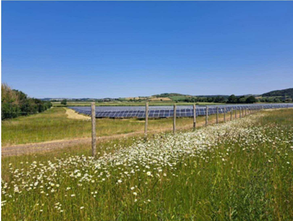
Plate 5: Typical Post and Wire Security Fencing
