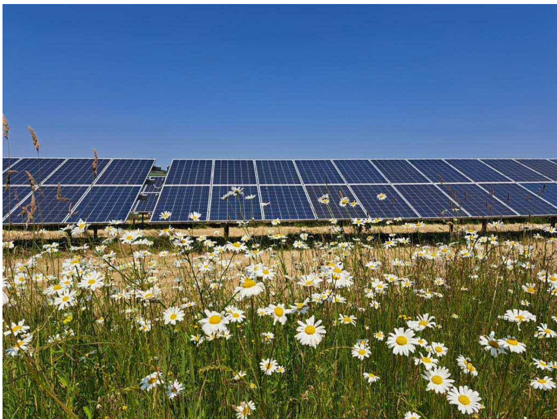
Plate 2: Typical Solar Panel Arrangement –Portrait Formation
